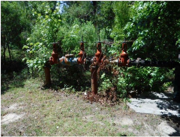
27. Backflow prevention device on the south side of the north detention basin
