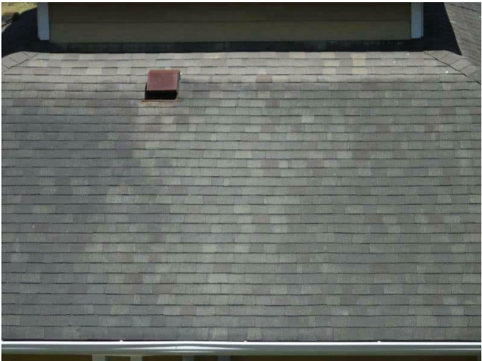
70. Typical asphalt composition architectural shingle roof
