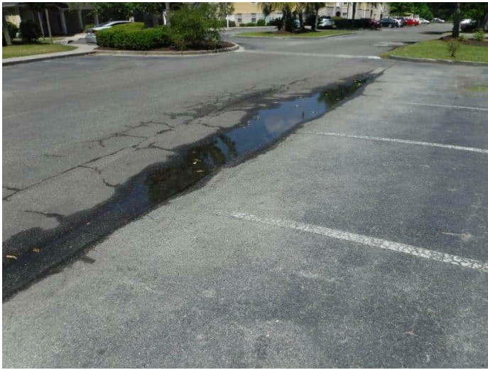
117. Ponding in the north drive aisle
