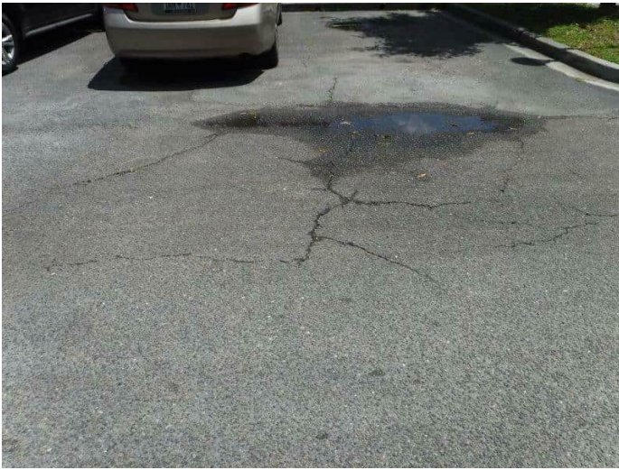
129. Linear cracking in the south drive aisle
