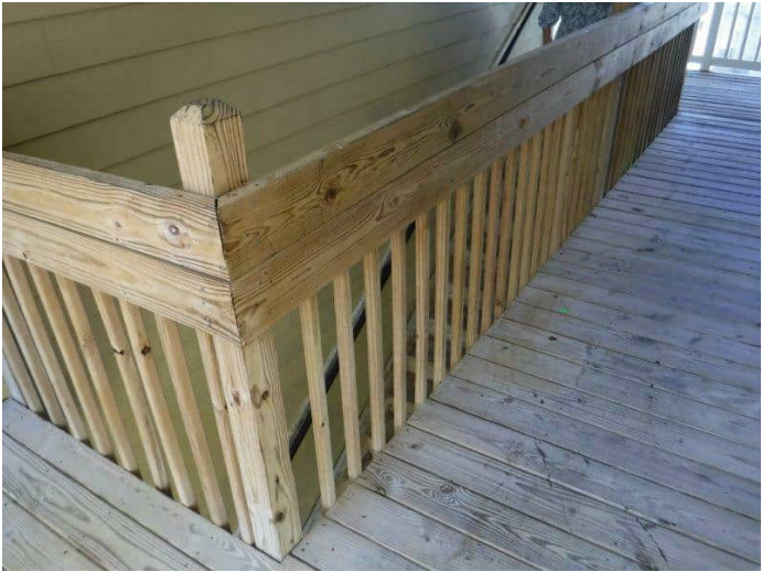
62. Typical stair guardrail
