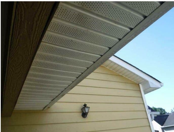
65. Typical vinyl soffit
