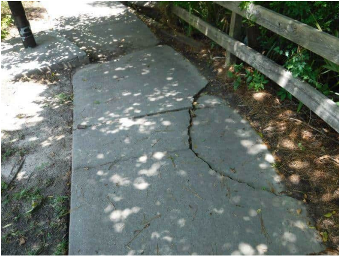
122. Cracked flatwork near the backflow prevention device
