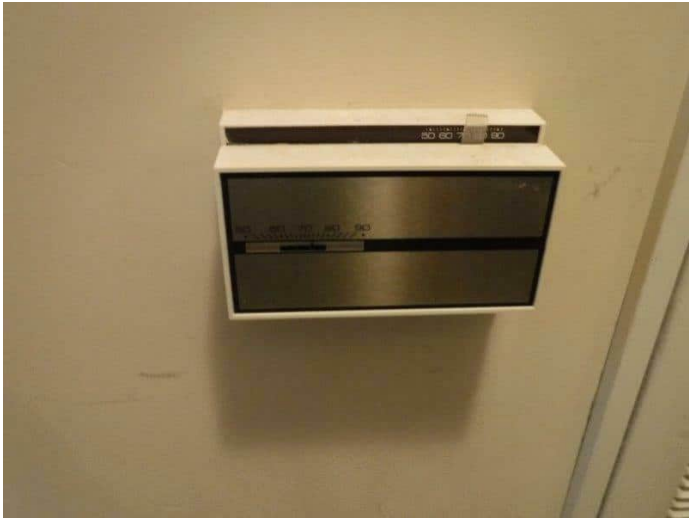
103. Older mercury thermostat in Unit 402
