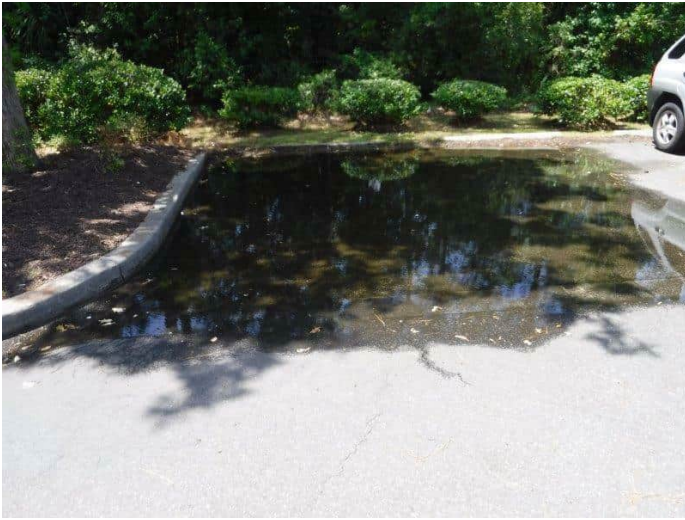
131. Ponding in the south drive aisle by Building 100
