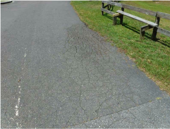
127. Alligator cracking in the west drive aisle
