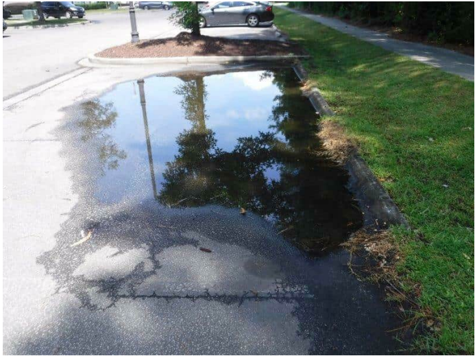
116. Ponding in the north drive aisle
