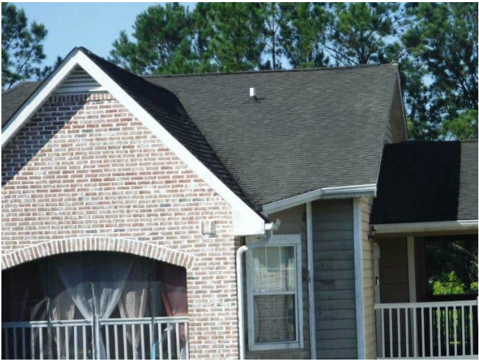
64. Typical asphalt composition architectural shingle roof
