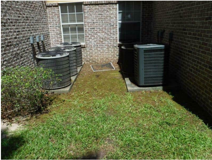
91. Older Payne condenser units with a newer Goodman unit
