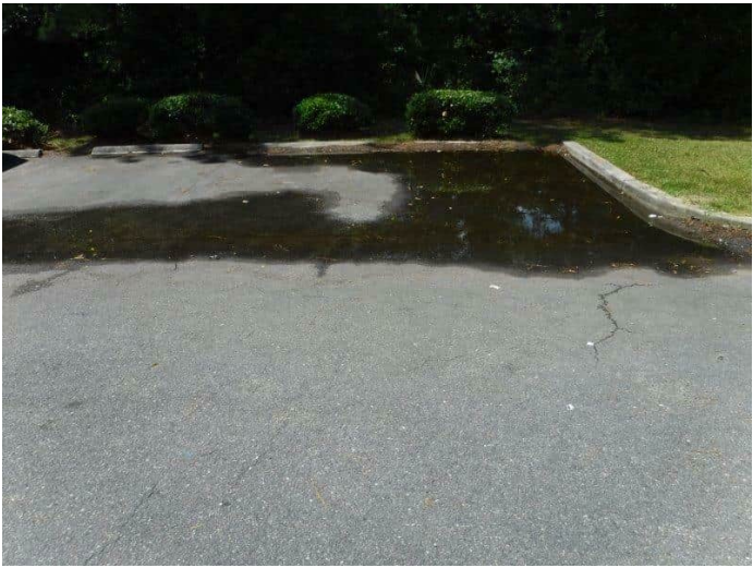
130. Ponding in the south drive aisle by Building 100
