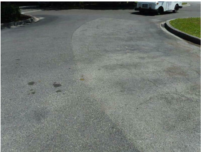
114. Typical asphalt pavement with minor linear cracking
