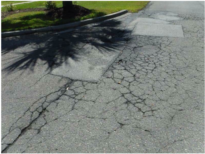
118. Alligator cracking at the entry drive aisle near the clubhouse
