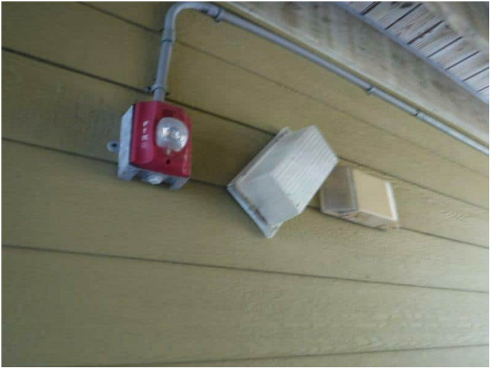
74. Typical alarm/strobe and lighting
