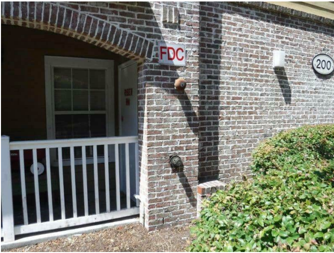
88. Typical fire department connection
